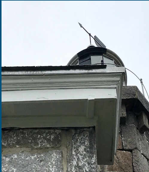
Proper gutters for roof drainage
