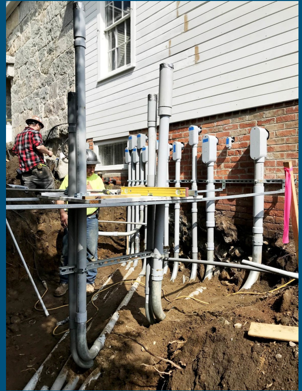
Instillation of new electrical systems
