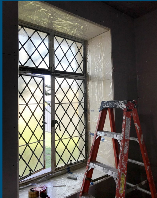
Weatherized windows to protect from the elements
