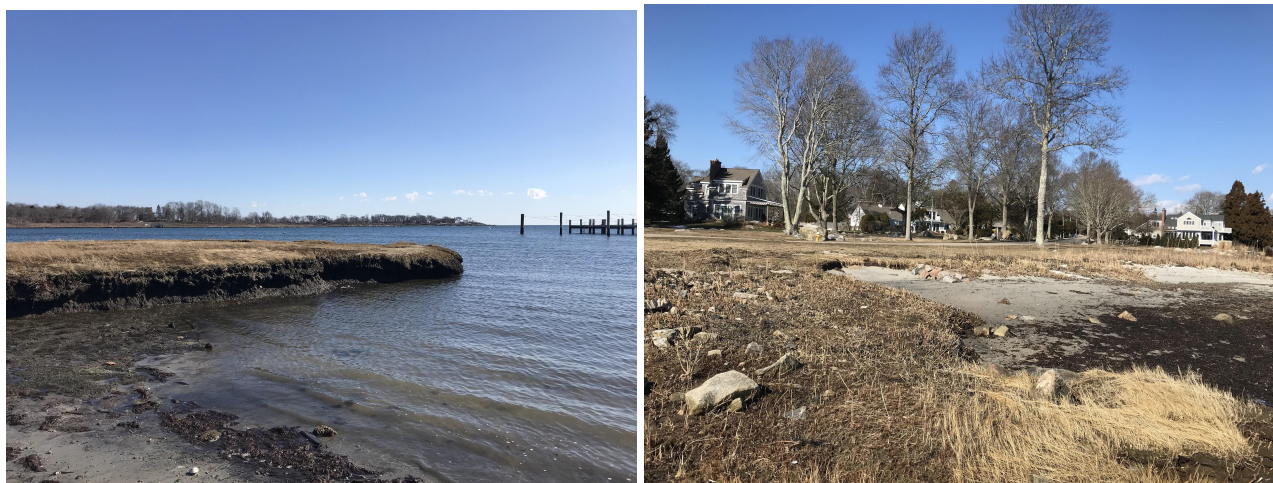
Pictures 4 and 5: The erosion and undercutting of the marsh adjacent to Chippechaug Trail. Note the rocks on the shoreline in picture 5 (right), which were placed by the residents of the island in an attempt to protect the shoreline from storm waves.
