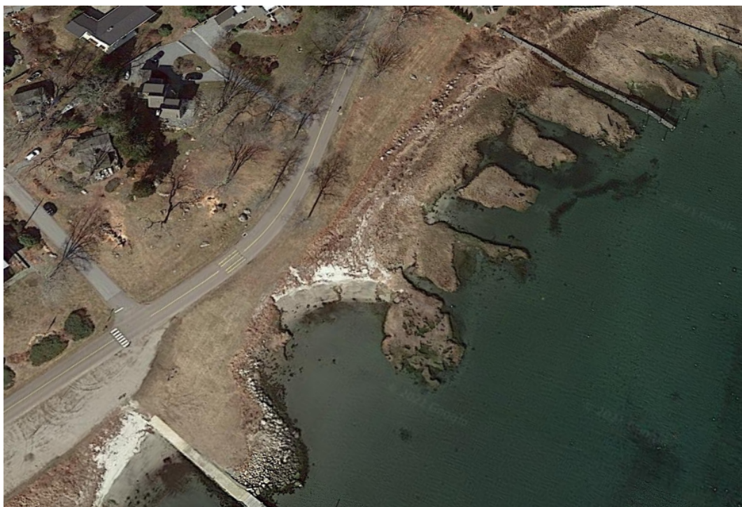
Picture 1: Aerial view of the portion of Chippechaug Trail closest to the eroding marsh.
